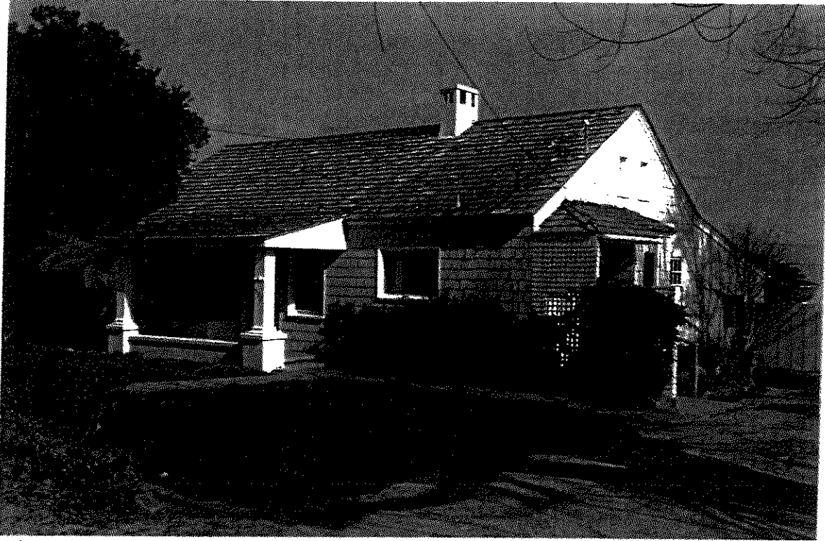
Photo #1. Looking NW at the south facing facade & east side-elevation, March, 2013.
